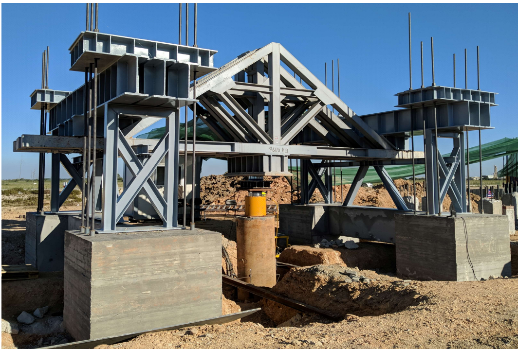
Figure 21- Bored Pile is Static Load test
