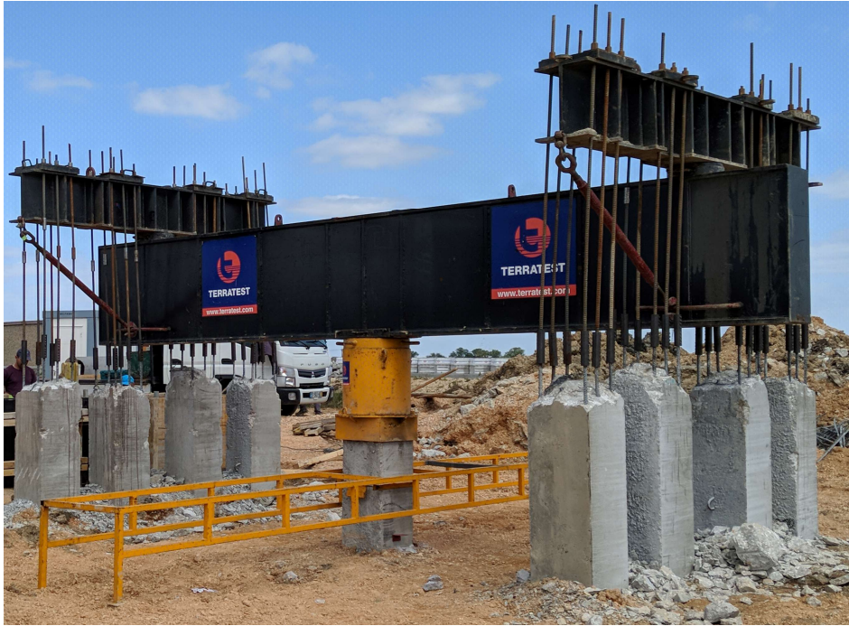
Figure 33- Static Load Test Performed on the Driven Pile.
